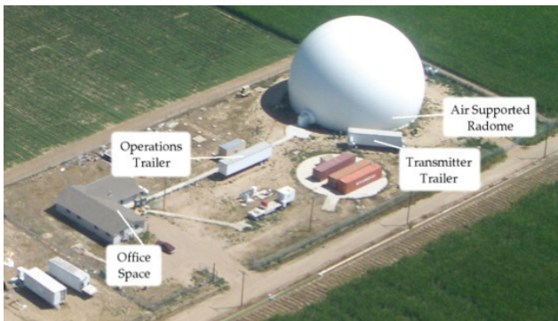
FIGURE 1. CSU-CHILL radar facility, with labels indicating major features.
