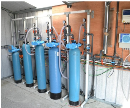
Figures 6(a) and (b) – The tertiary treatment system installed at the WRF and the HMI installed at the WRF.
