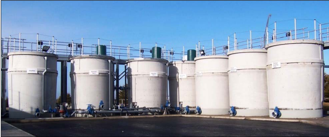
Figure 4 - Photograph of the PFBR at the WRF. Shown from right to left are; 1 No. sludge holding tank, 2 No. primary settlement tanks, 1 No. balance tank, 2 No. reactor tanks, and 1 No. clarifier.
