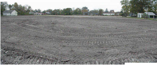
Figure 5 Completed Demolition and Site Clearance Phases
