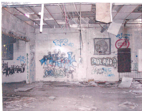
Figure 2 Inside of Old Factory Building
