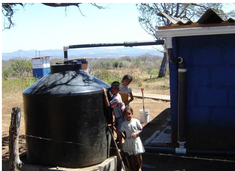
FIGURE 2 NICARAGUA I: RAINWATER CATCHMENT SYSTEM
