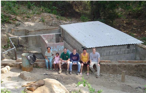
FIGURE 4 EL SALVADOR WATER STORAGE TANK
